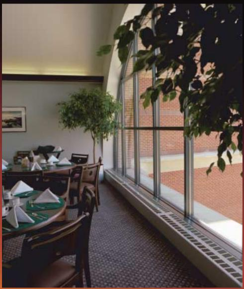
Hydronic Finned-Tube Radiation
